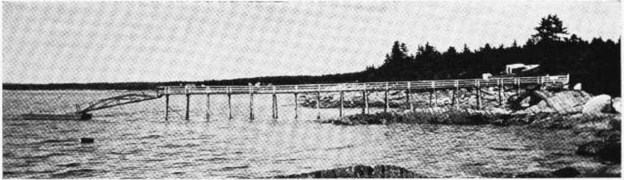
Float and runway (destroyed) — to be relocated and rebuilt by the Pemaquid Point Association
