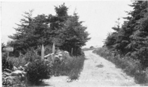
ROADWAY FROM HOTEL TO OCEAN
